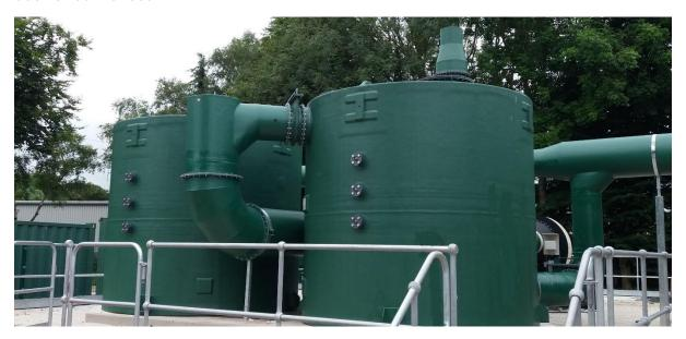
One recent project highlights this expertise: Roperhurst designed and installed a multistage wet scrubber system for a large municipal wastewater treatment plant in the South of England. The system was built using PVCu and GRP components to resist the corrosive effects of hydrogen sulphide and organic acids. Not only did the project
